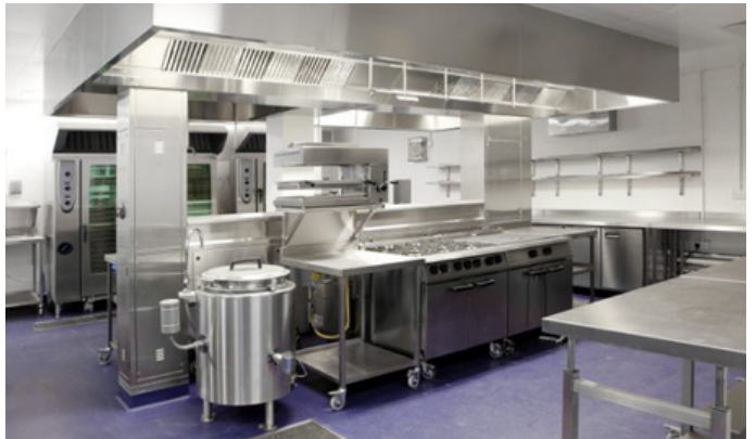
GALLEY, LAUNDRY & ACCOMODATION
